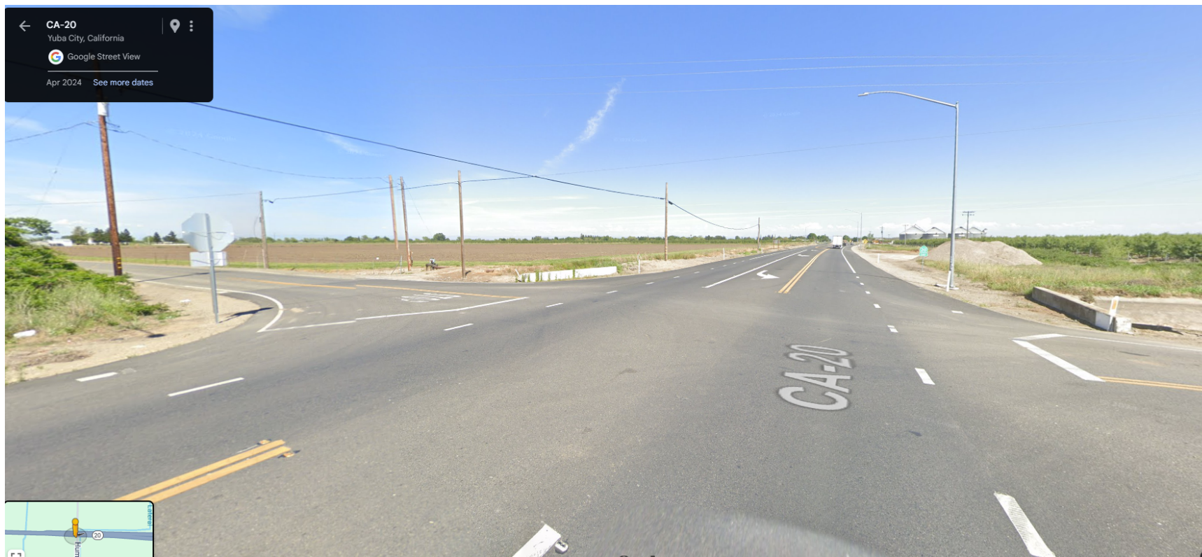
Figure 4: Streetview looking east on State Route 20 and north leg of Humphrey Road
