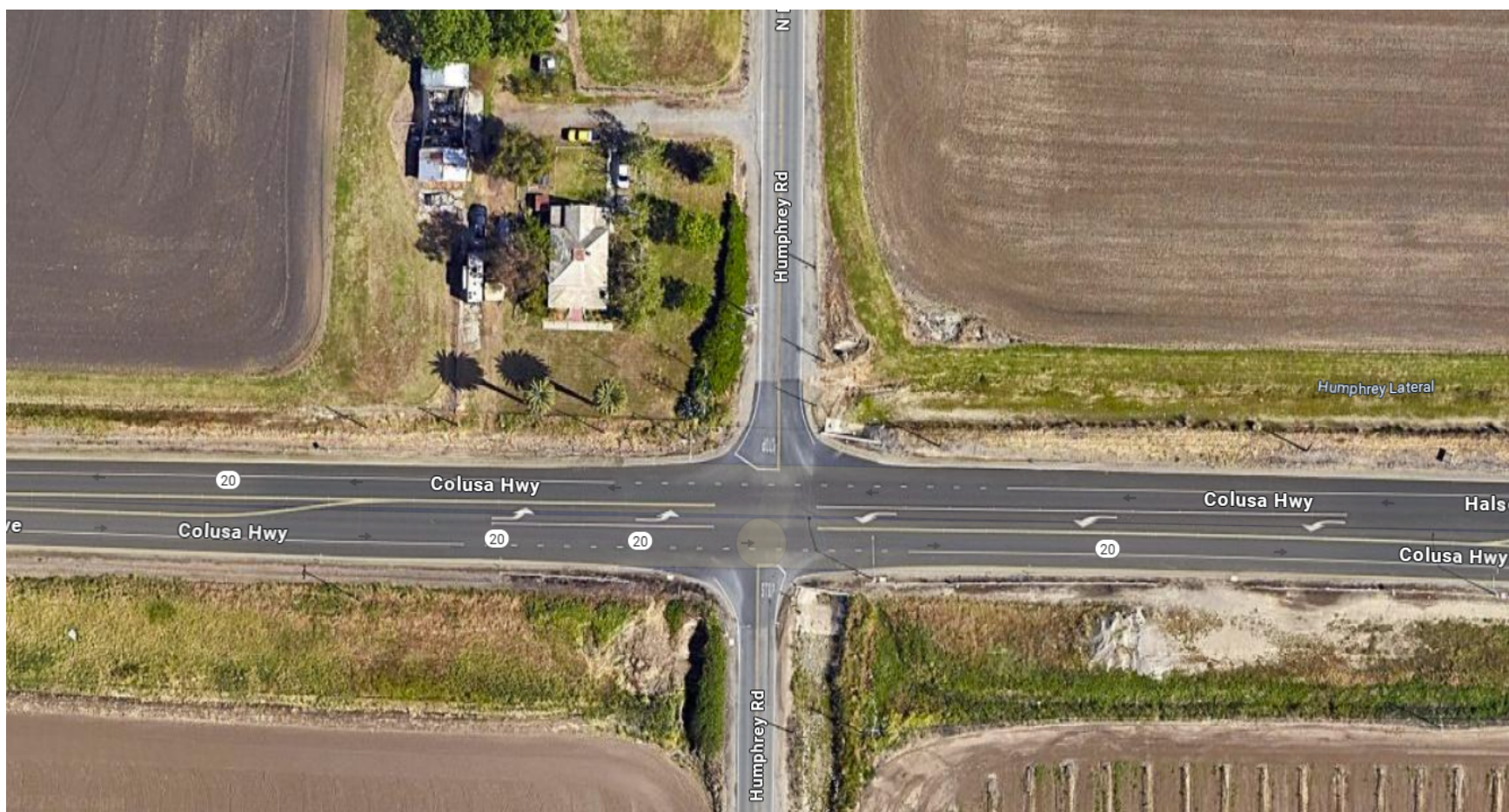
Figure 2: Aerial view of State Route 20/Humphrey Road Intersection
