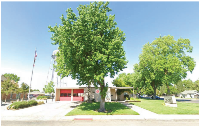
Picture of Yuba City Fire station at 824 Clark Avenue.
