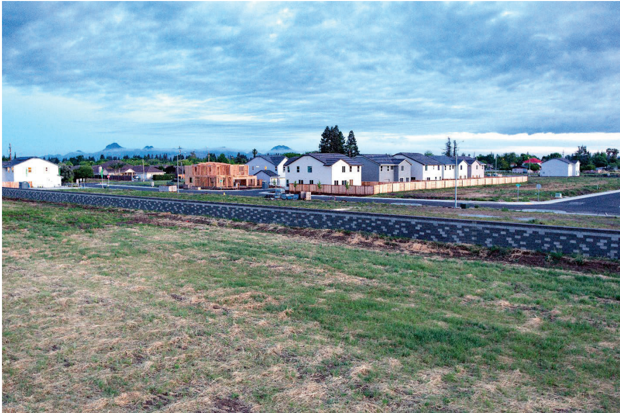
View of subdivision under construction with vacant field in foreground.
