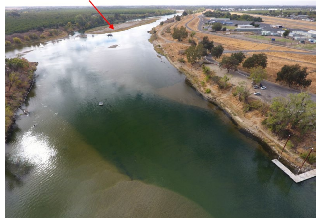
Figure 2: Sediment Deposited South of the Confluence of the Feather and the Yuba Rivers that will be Dredged in Phase 2
